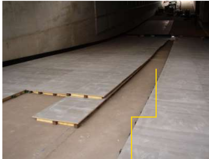
Installation from sides towards tolerance zone
