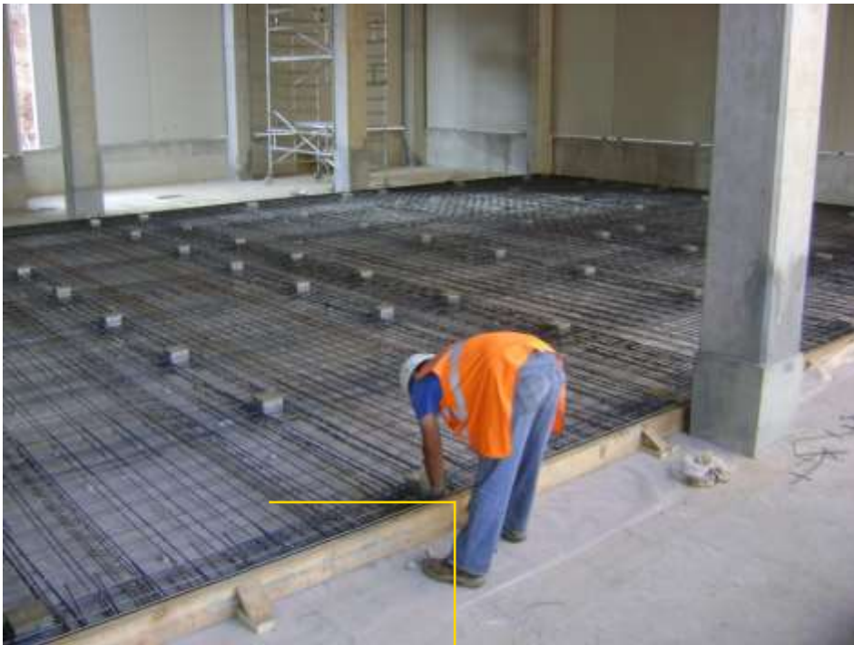
Reinforcement grid (double layer) installed
