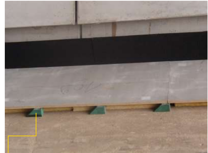
Conical pads to create enough load bearing surface
