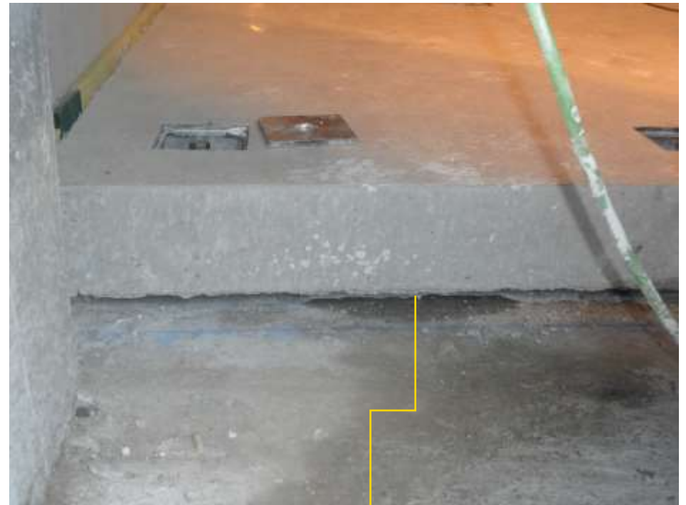
Floating floor jacked up
