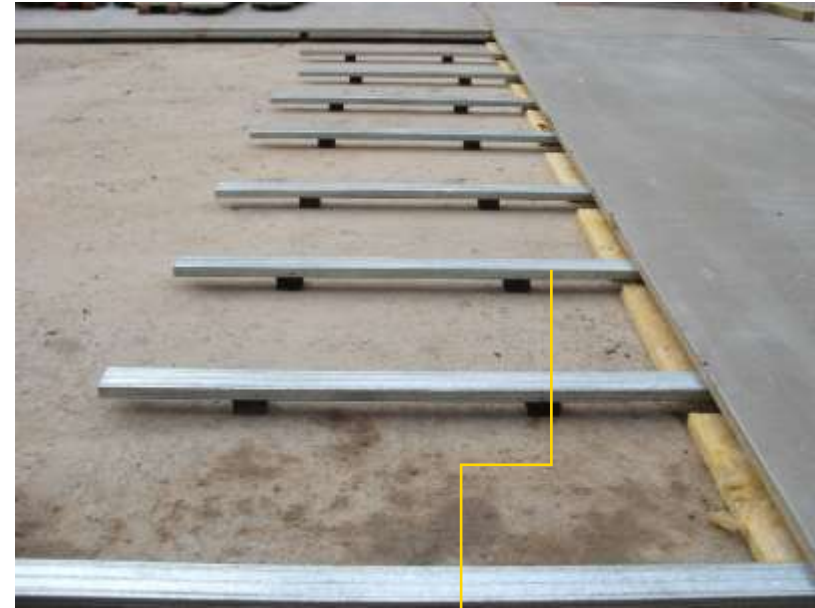
Lost formwork for floating slab concreting
