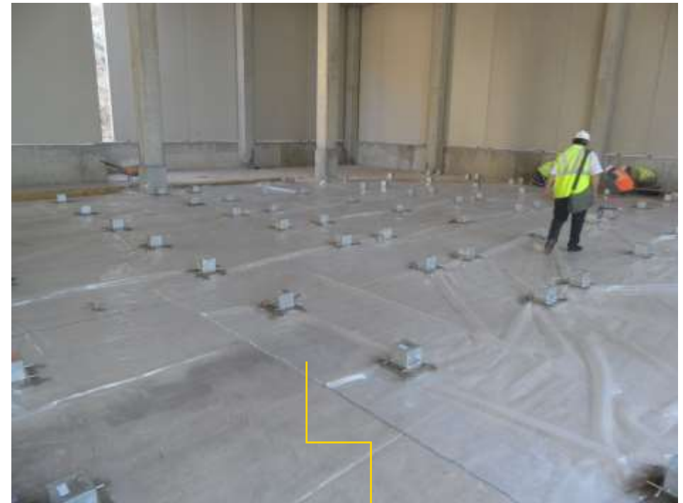
PE foil on structural slab + taped around boxes
