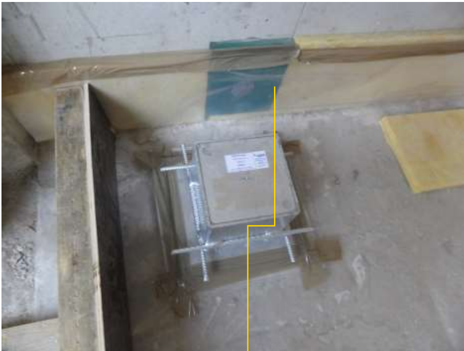
Installation of perimeter isolation and lateral buffers
