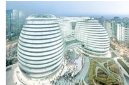
Galaxy Soho Office Building, Beijing (China)
